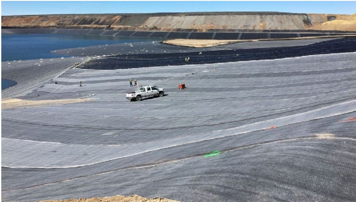
Figure 4. Photo Illustrating the Development of a Tailings Storage Facility with a Lining System 6
